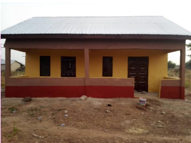
Figure 4.2: Constructed Shea Processing Centre at Zugu
